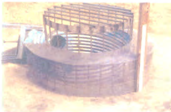
Figure 1 Example of Extended Detention Outlet Structure
