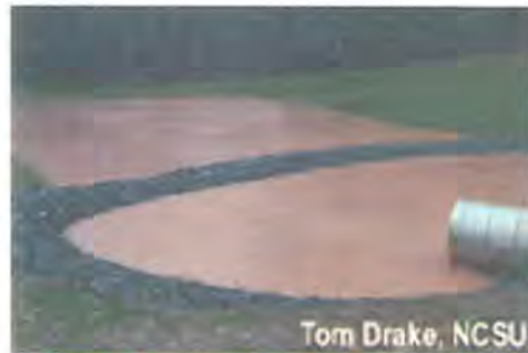
Figure 2: Forebay filled with storm water
