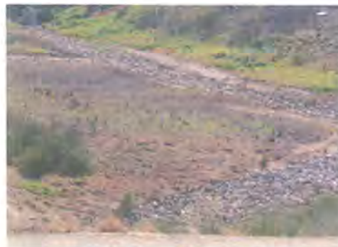
Figure 3: Gravel filled low-flow trench
