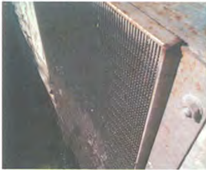
Trash rack with screen
