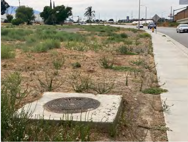
Photo 7 Sewer at northwest end of NWC lot
